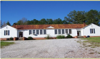
Woodworking Education Center 10544 Hwy 17, Maylene, AL 35114
